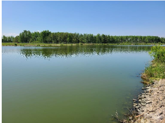
A picture of one of the lagoons at the Village's WWTF. Wastewater is treated in these ponds and then discharged to the Pokegama River per the Village's discharge permit.
