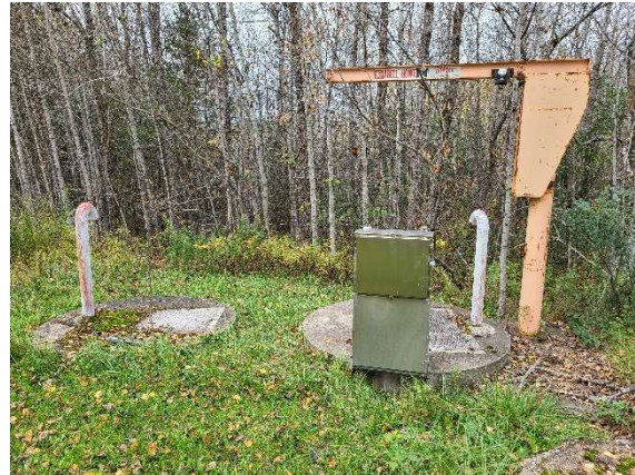
A picture of the Village's Lift Station wet well and valve vault. Upgrades to the Lift Station are included as part of the recommended alternative.
