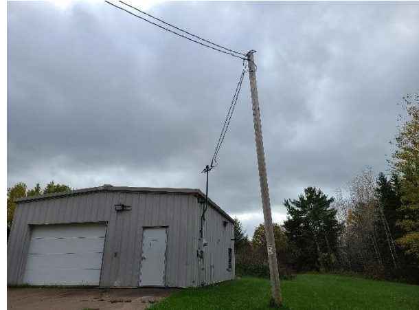
Shown is a picture of the maintenance station. SWLP recommends that the electrical service should be upgraded.
